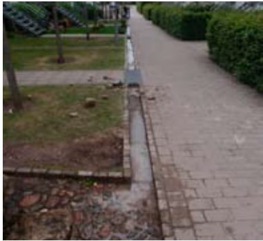
Abb. 4.62: Hannover, Kronsberg, Wasserrinne
